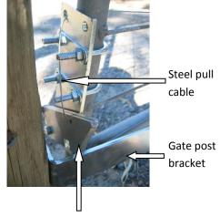
Gate flipper plate pulled up by steel cable attached to gate motor swing arm
